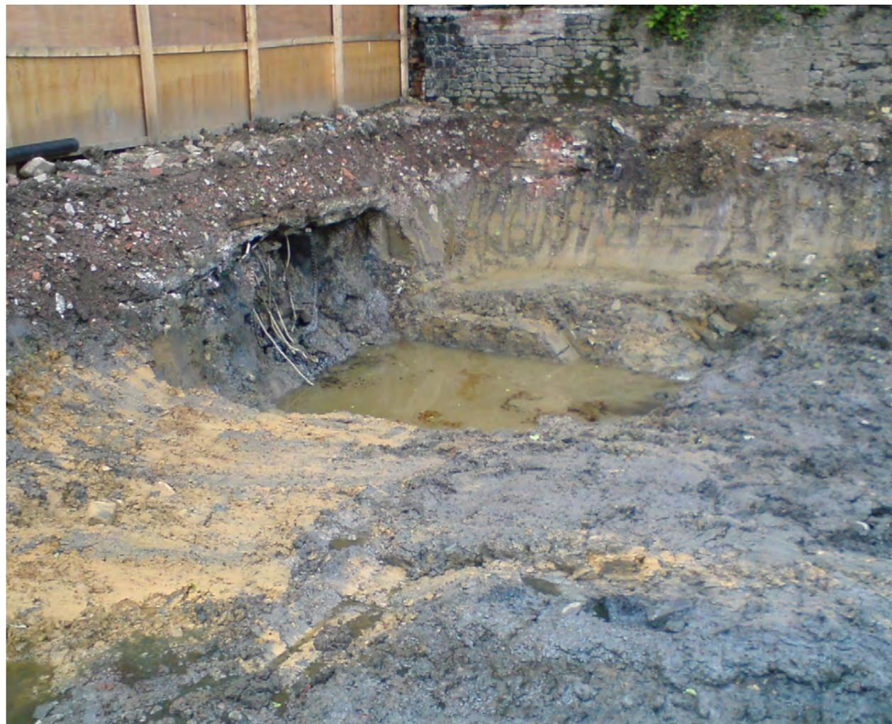
An excavation shows soil contamination at an industrial site in England. In the early 2000s, researchers developed a method to smolder hazardous organic liquids such as oils, solvents, and coal tars that were found in the soil.
